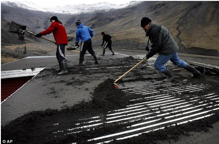
Clearing basaltic tephra from roof, Iceland
